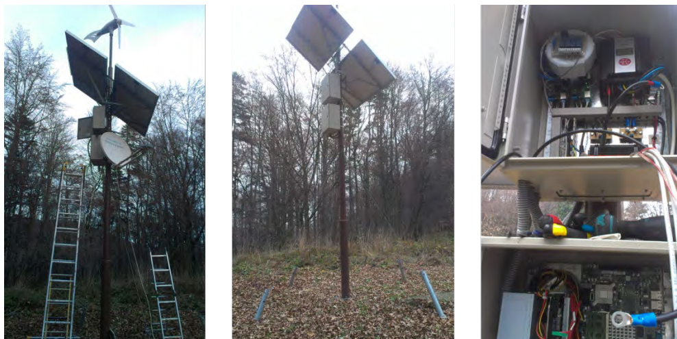
Obr. 6 Kamerový systém a príslušenstvo Fig. 6 Camera system and its equipment
