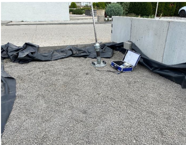
Obr. 8. Situácia parkoviska S_{21} , zdroj NARA-SK Fig. 8. Situation of parking lot S_{21} , source NARA-SK
